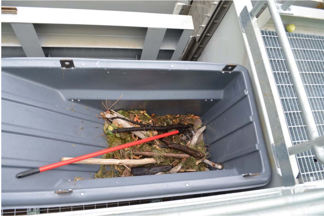
Figure 4-11 - Type of Debris Removed at the North Fork FSC Coarse Debris Rack
